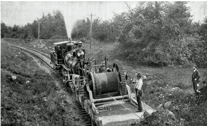
ABOVE LEFT: Locomotive coupled to a Lidgerwood Unloader to provide steam power for the winch drive.
