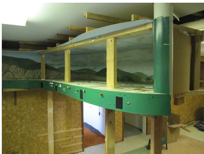
ABOVE: Brian Pate's basement showing the Dawson City section stripped of fascia, base and structures.
