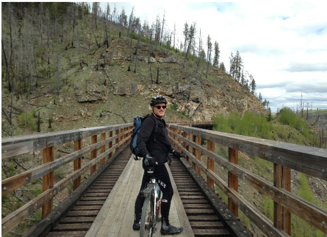
ABOVE: Your intrepid reporter on wood trestle no. 4. At 150x37 metres, it is the longest and tallest of the wooden trestles and third in height after the Pooley and KLO Creek steel trestles.
