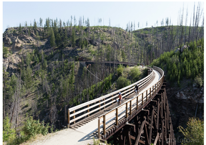
ABOVE: Wood trestle no. 8 (foreground) 73x21 and steel trestle no. 9 (KLO Creek) 111x48 in the background (dimensions in metres).
