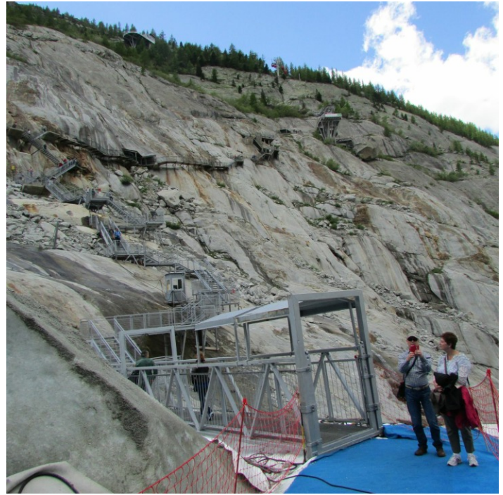
ABOVE: Engineered walkway from the gondola base to the ice caves elevation seen from the bottom.
