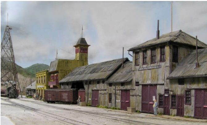
ABOVE: Train 401 enters Dawson City through the legs of the ferry tower
