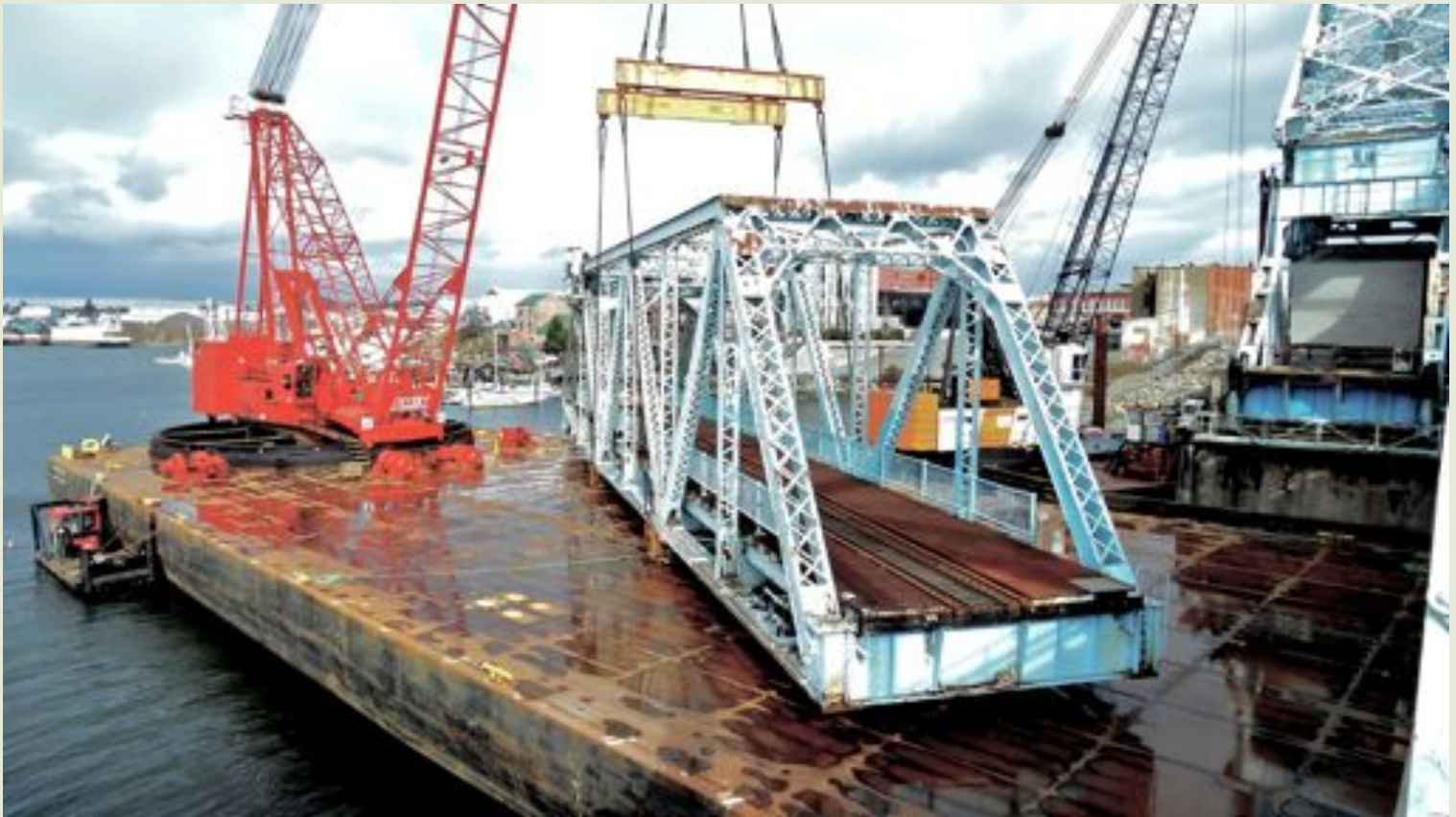
Johnson Street Bridge Removal
